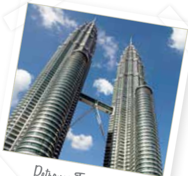
Petronas Twin Towers
